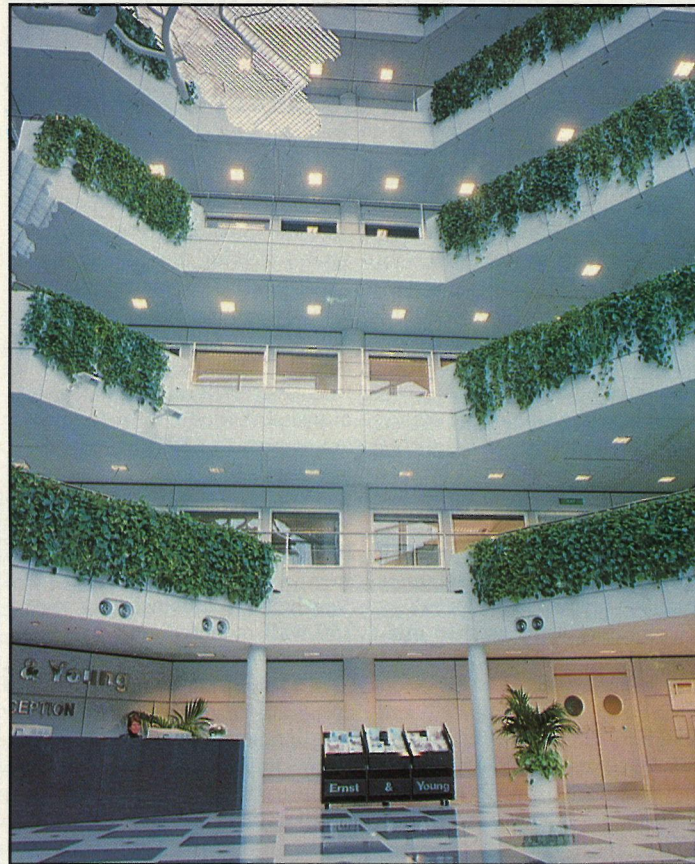
Compact luminaires used in the atrium at Bristol's Bridewell House.
